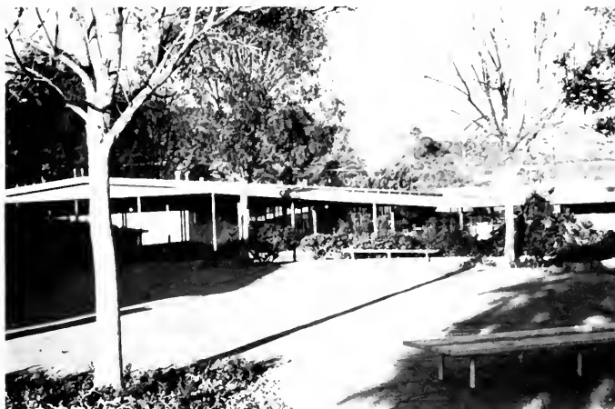
Photo 13. Fenton Avenue Elementary School. Essentially no damage.
